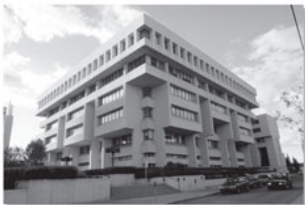
Then and Now The first courthouse in the Canadian Northwest (top) and the current Edmonton Law Courts (bottom).
